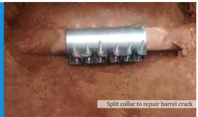
Mechanical joint in supply pipeline
