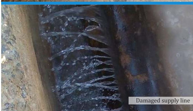
Mechanical joint in supply pipeline
