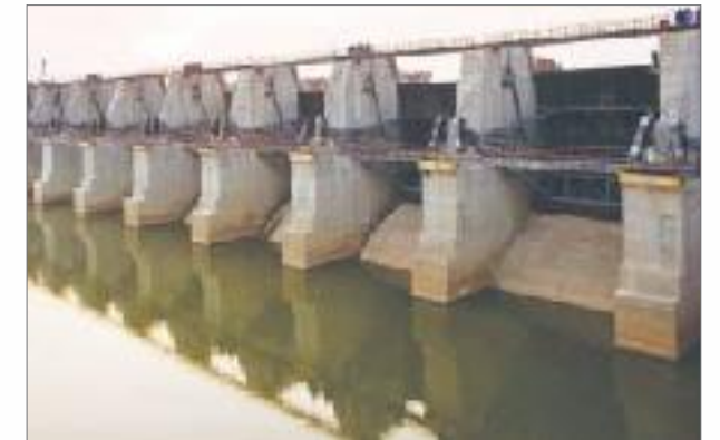
Hydro Mechanical Work, Gosikhurd Barrage, Maharashtra
