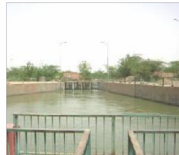
Rajiv Gandhi lift Canal in Rajasthan
