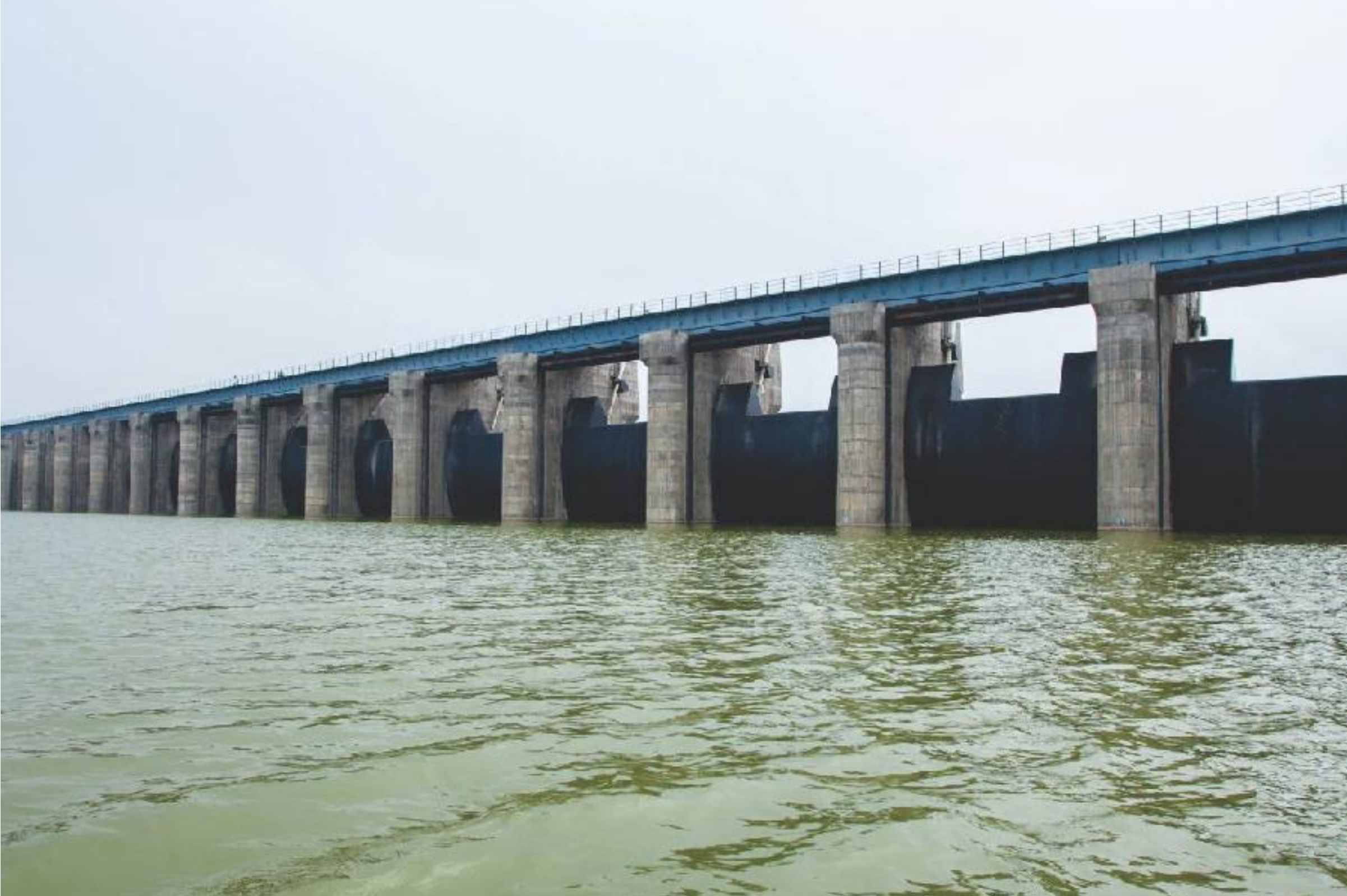
Concrete Gravity Dam, Kalisindh, Rajasthan
