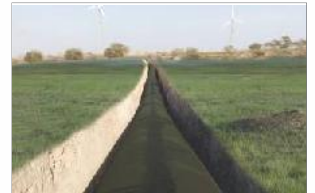
3000 MM Dia MS Pipeline, Sauni Yojana, Gujarat
