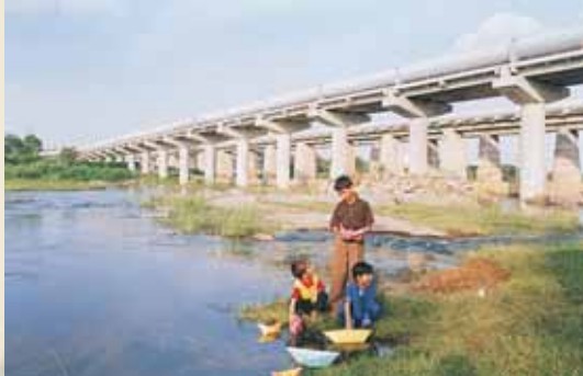
Cauvery Water Supply Project
